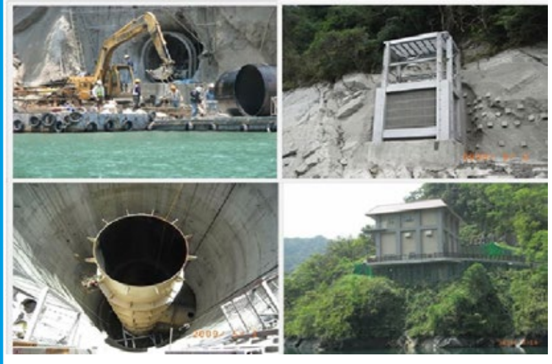
Figure 8 Stratified water intake shaft during construction, completed in 2009 (Photos taken from http://wcis.pcc.gov.tw/ )
