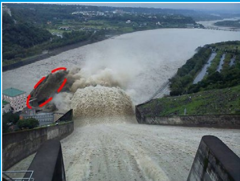
Figure 10 Sediment sluicing after power plant water intake tunnel renovation (Photo taken from http://www.wra.gov.tw )
